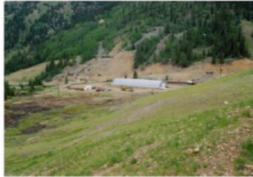
American Tunnel, 1998, (after) – SGC removed 80,000 tons of mostly historic mine waste and tails.
